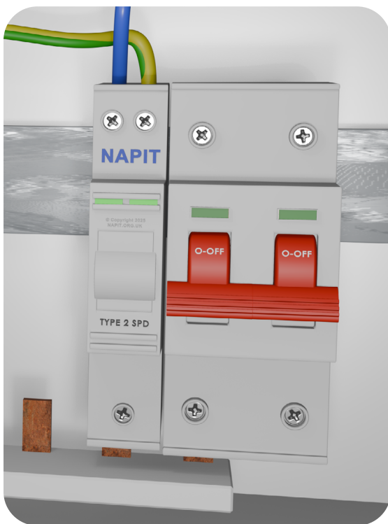
Fig 1. SPD installed directly onto the busbar and protected by the DNO cut-out fuse
