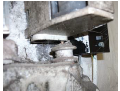
Visible bare wires
